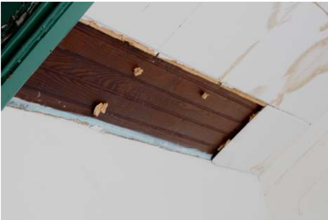
Original bead board under acoustical tiles, under stairs to third floor, 2015.
