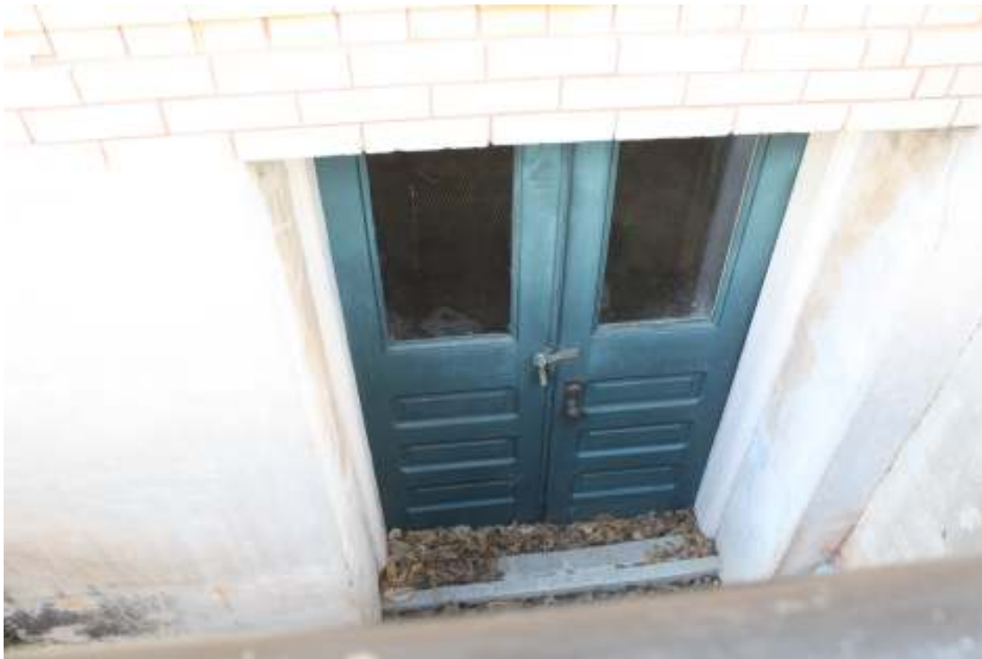
Glass-and-wood-paneled doors that open to the basement from the sidewalk on West Main Street, 2015.
