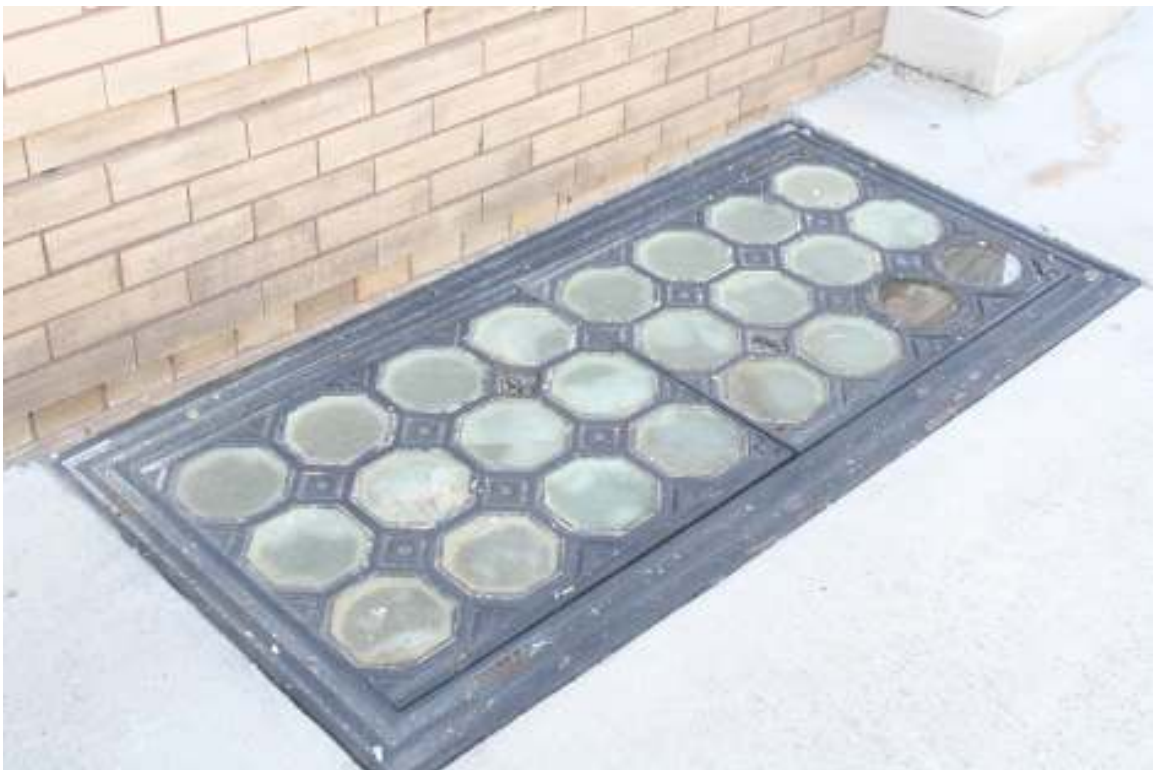
Octagonal glass-block sidewalk grate, West Main Street, 2015.
