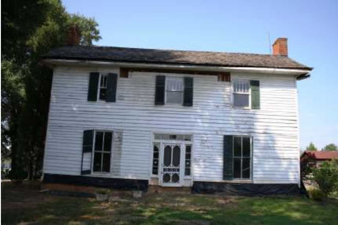
House, 2013. East elevation, camera facing east. Showing facade after removal of two-story porch dating from the 1950s.
