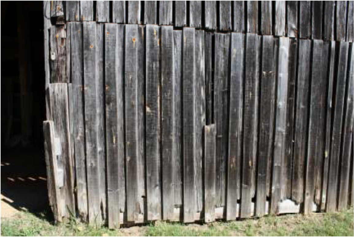
West Elevation. Board-and-batten siding.
