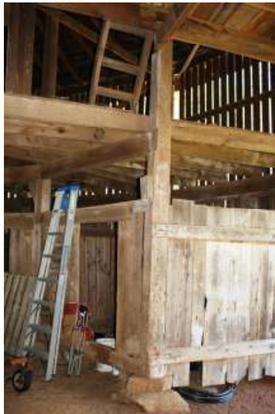
East Elevation, first floor. Large supporting beams are hewn and the lesser ones are sawn.
