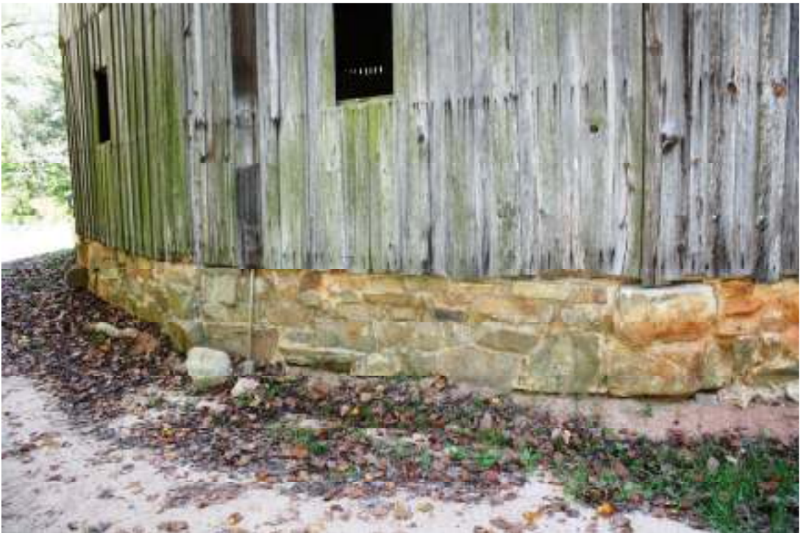
North Elevation. Visible is the rock foundation, and board-and-batten siding and small openings to the first floor.
