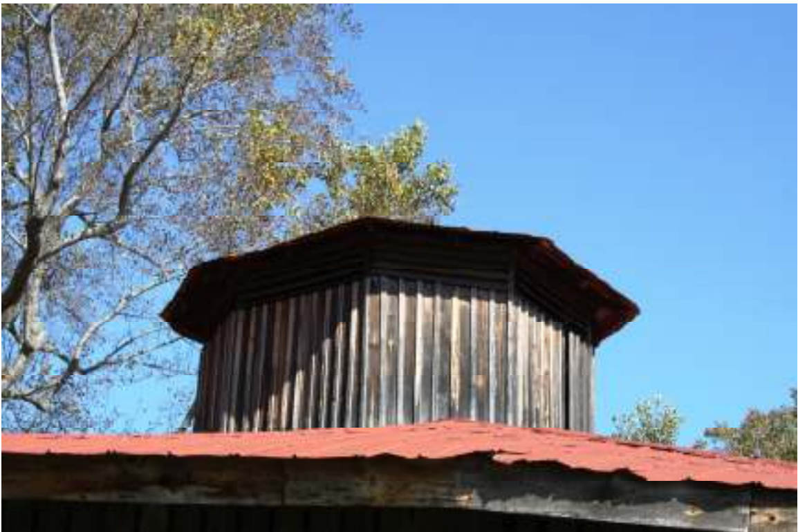
Eight-sided blind cupola from which a low, polygonal roof extends.
