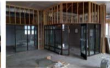
Framing - interior storefront installed
